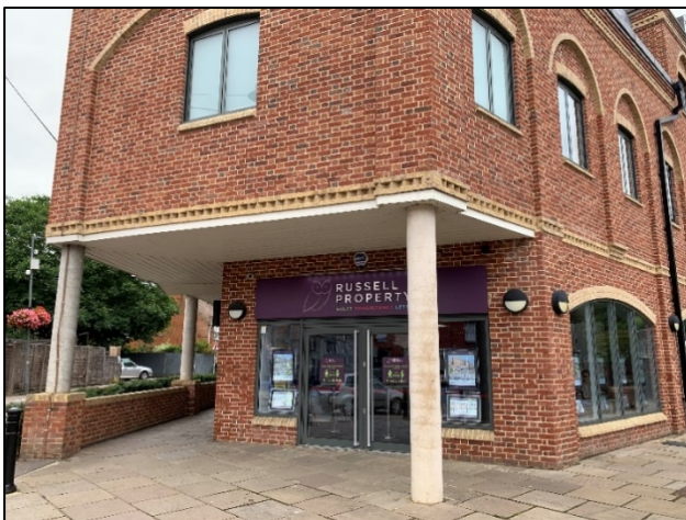
Modern development, Lower Street
